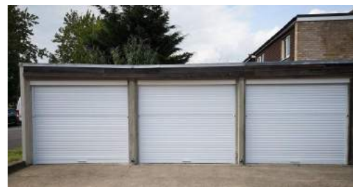
Doors replaced with Roller Shutter Doors
